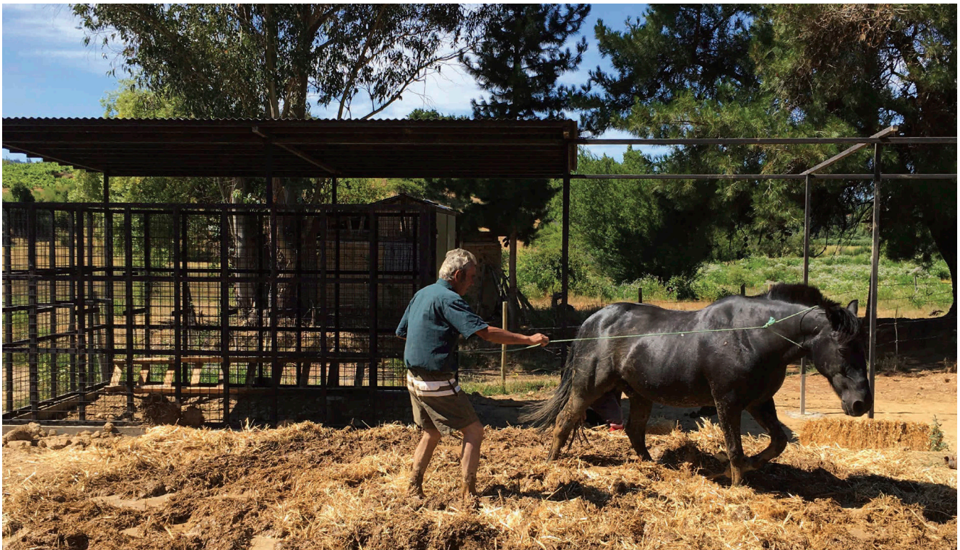
Figure 1. The preparation mixture of silt, clay, straw, and water for the construction of the “Techno-Quincha.” The materials are mixed using mares to ensure a homogeneous mixture. The Authors
